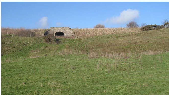
Leven and East of Fife Railway: an embankment and bridge on the trackbed of the Leven and East of Fife Railway at Newark. The railway left the coast here for a more inland route behind St Monans and Pittenweem.
